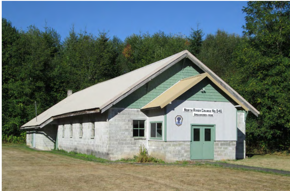
Figure 5.12: North River #946 in Pacific County (Example of an enclosed vestibule on a purpose-built hall)
