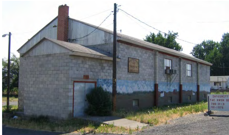
Figure 5.21: Buena Vista #415 in Benton County (Example of concrete block building)
