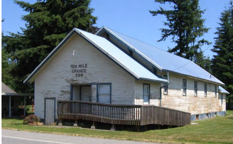
Figure 5.20: Ten Mile #399 in Whatcom County (Example of frame building with clapboard cladding)
