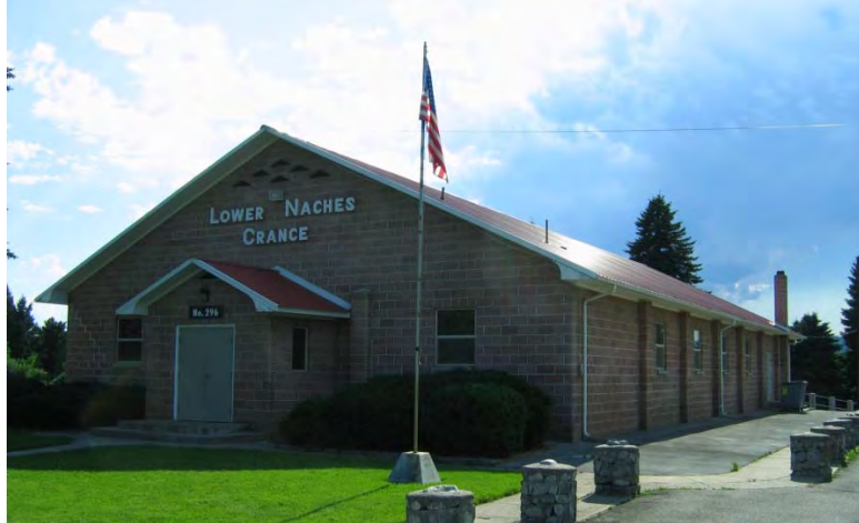
Figure 5.23: Lower Naches #296 Yakima County (Example of traditional elongated rectangle form reproduced using new materials – concrete block, in this case)
