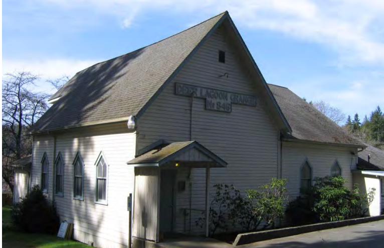
Figure 5.32: Deer Lagoon #846 in Island County (Example of peaked side windows characteristic of former churches adapted for use as grange halls)
