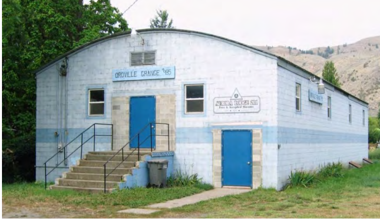
Figure 5.17: Oroville #985 in Okanogan County (Example of curved roof form)
