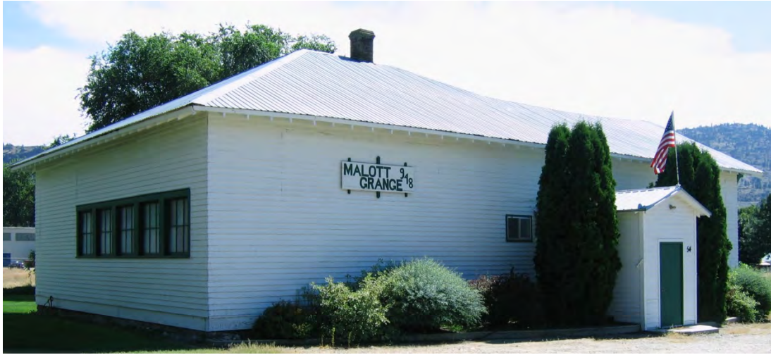
Figure 5.30: Malott #948 in Okanogan County (Example of window bank characteristic of former school buildings adapted for use as grange halls)
