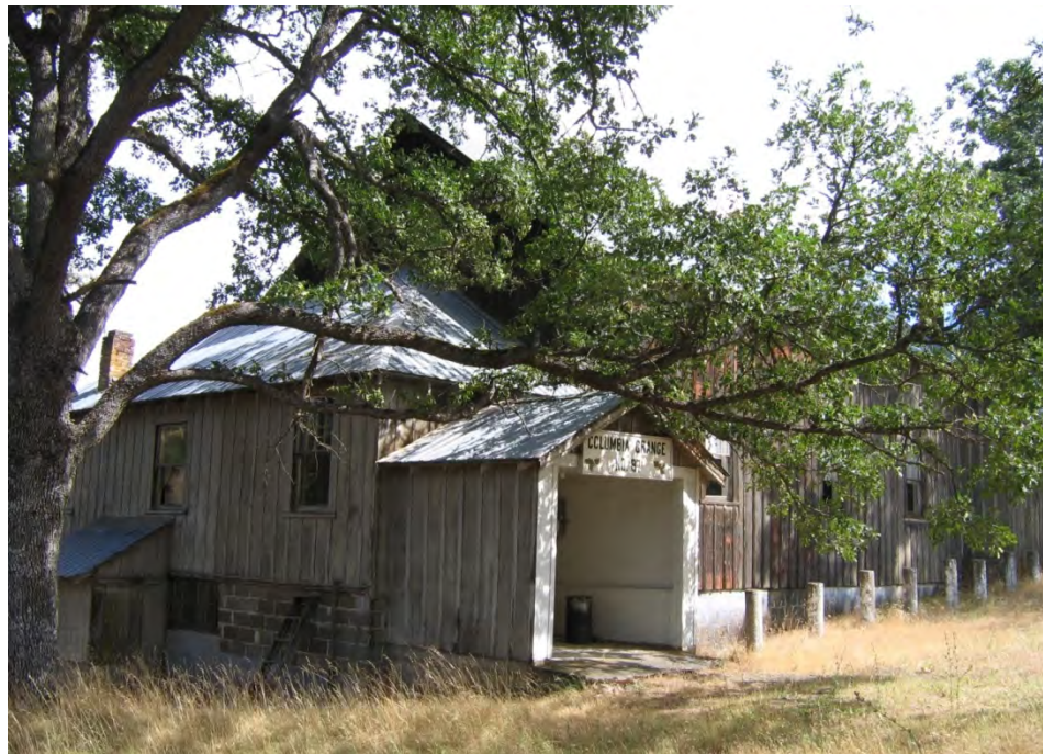
Figure 5.48: Columbia #87 in Klickitat County (Appears to be the oldest purpose-built grange hall in Washington State)
