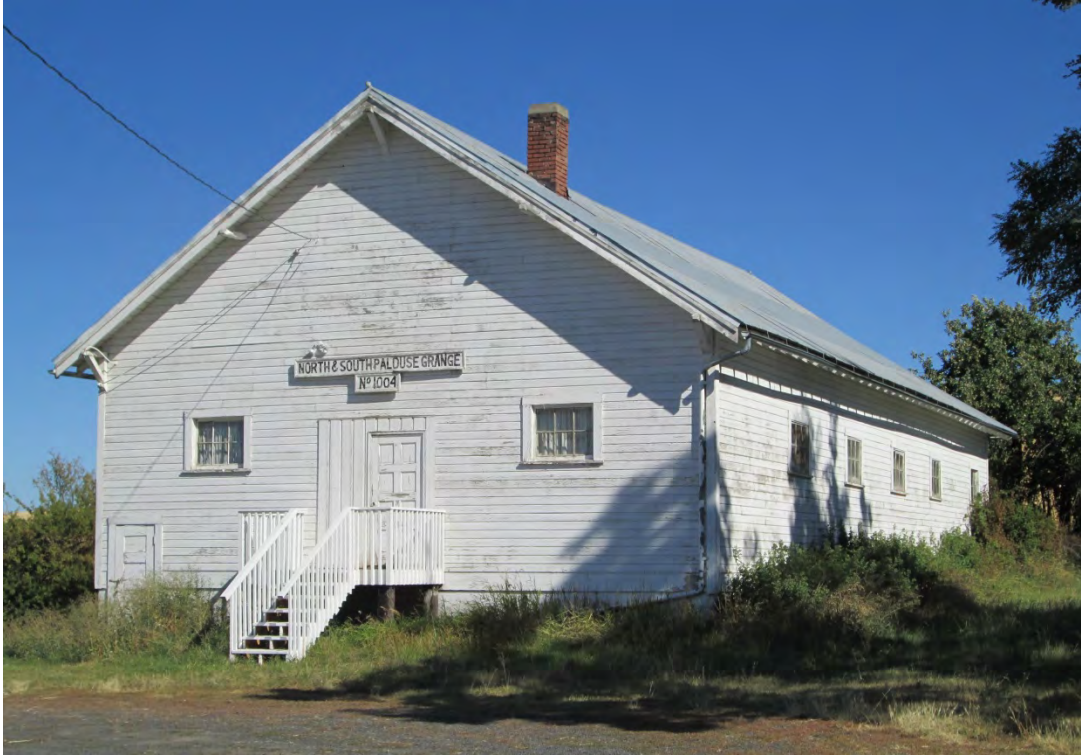
Figure 7.29: North & South Palouse #1004 in Whitman County
