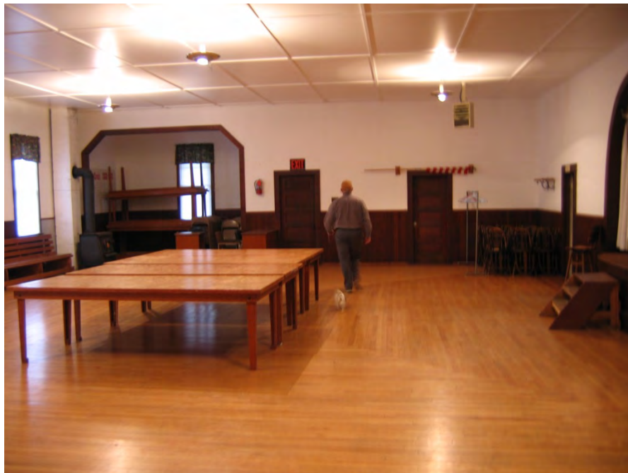
Figure 7.5: Lincoln Creek #407 in Lewis County (Example of interior with dropped ceiling)
