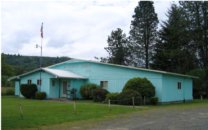
Figure 5.38: Mossyrock #355 in Lewis County (Example of a grange hall reconstructed from salvaged materials)
