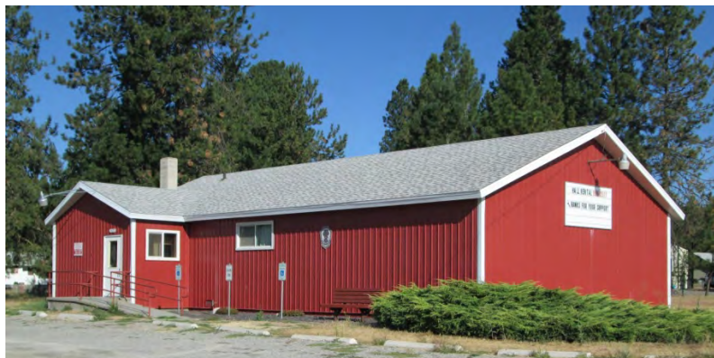
Figure 5.22: Tri-Community #1008 in Spokane County (Example of prefabricated metal building)
