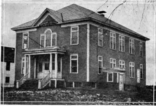
FIG. 34.—Grange Hall at Newbury, Mass.
