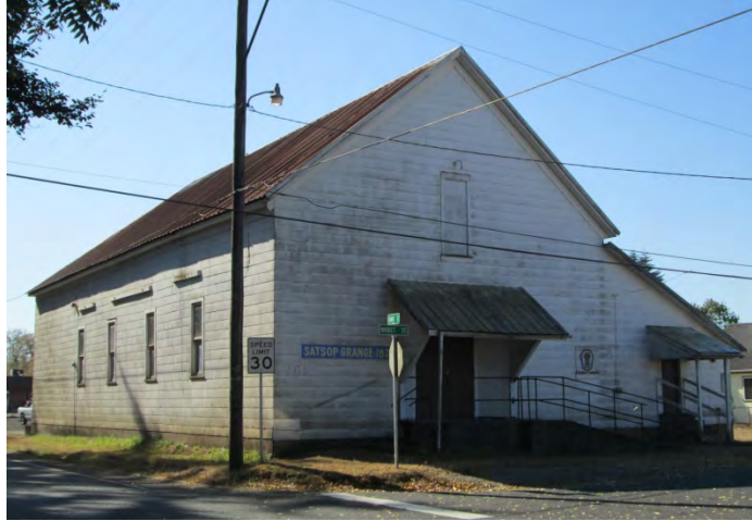
Figure 5.14: Satsop #183 in Grays Harbor County (Example of front gable form)
