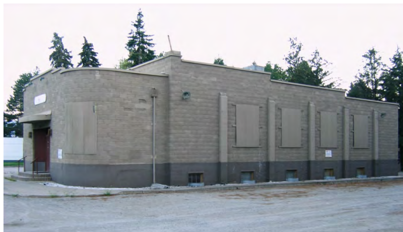
Figure 7.13: East Wenatchee #1012 in Douglas County (Windows covered to deter vandalism)
