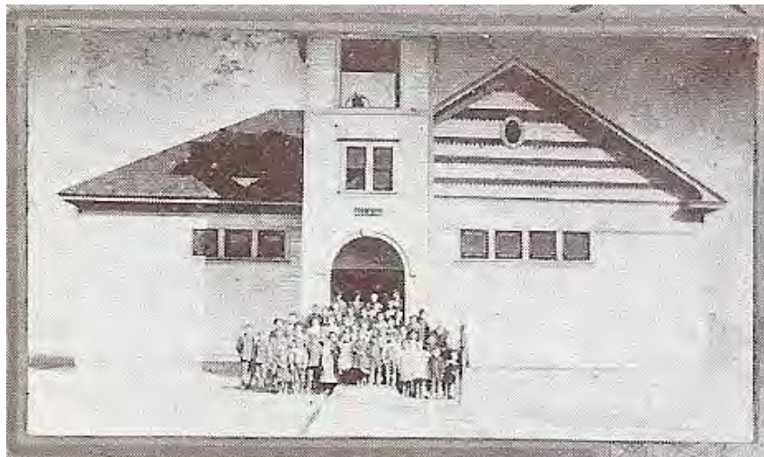
Figure 5.29: A school in Yakima County (1911), apparently built on the same plans as Half Moon School, now Half Moon Grange #907 (from Washington State Department of Education. Consolidation of Rural Schools and Transportation of Pupils . Olympia, WA: 1911, pp. 107)
