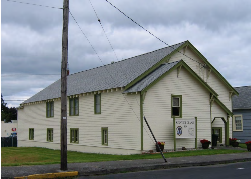
Figure 5.56: Sunnyside #129 in Cowlitz County (built in 1939)
